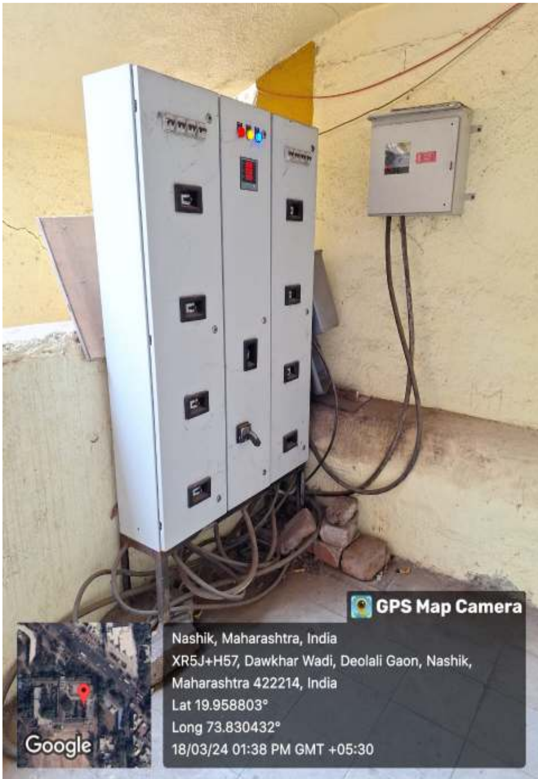
Wheeling of Grid
