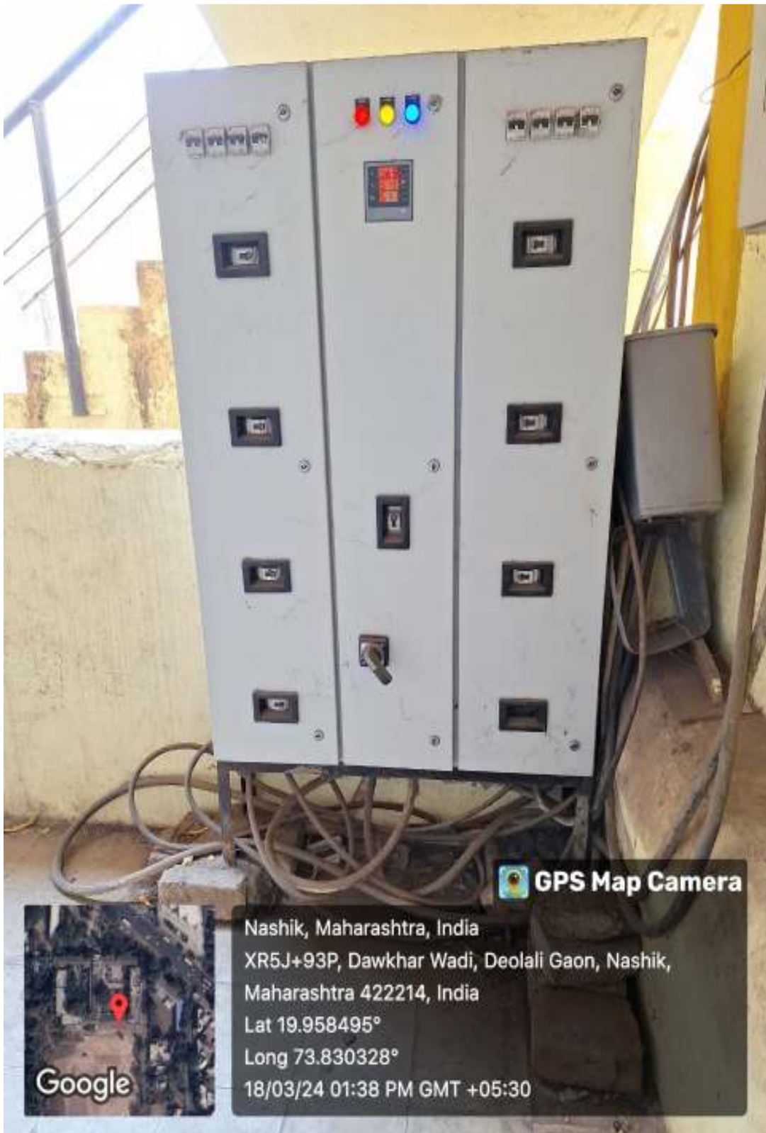
Wheeling of Grid
