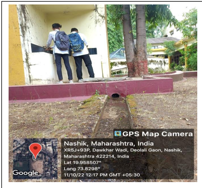
Waste water recycling
