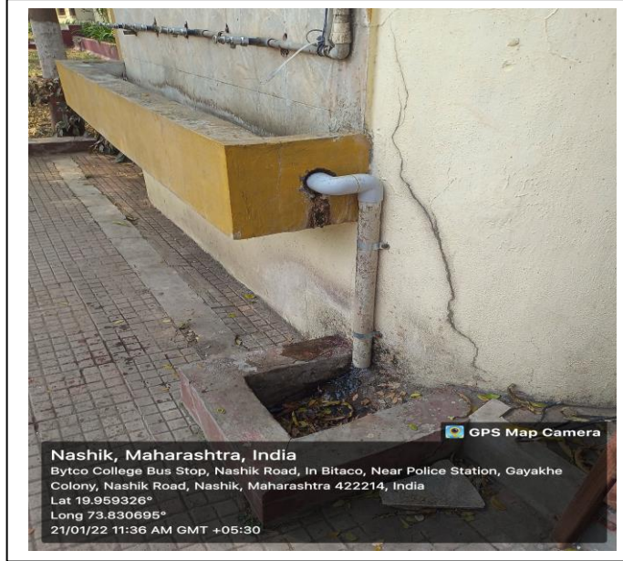
Waste water recycling
