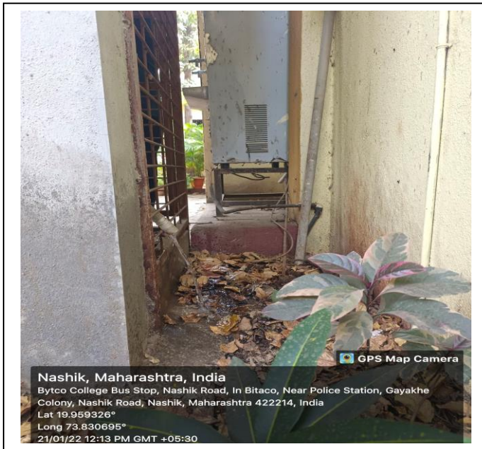
Waste water recycling
