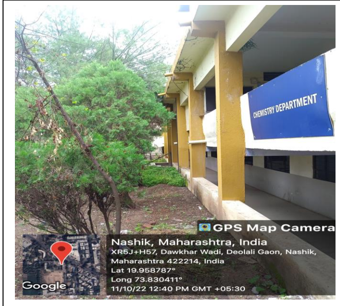
Waste water recycling
