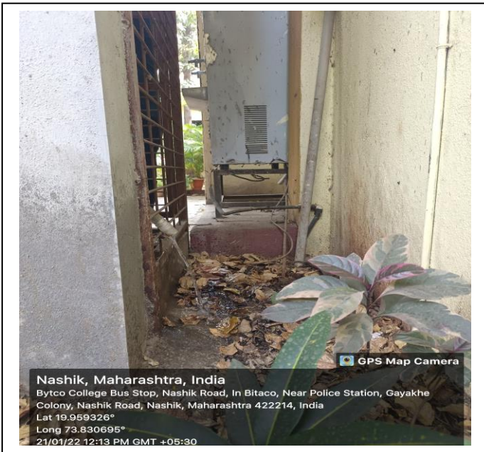
Waste water recycling
