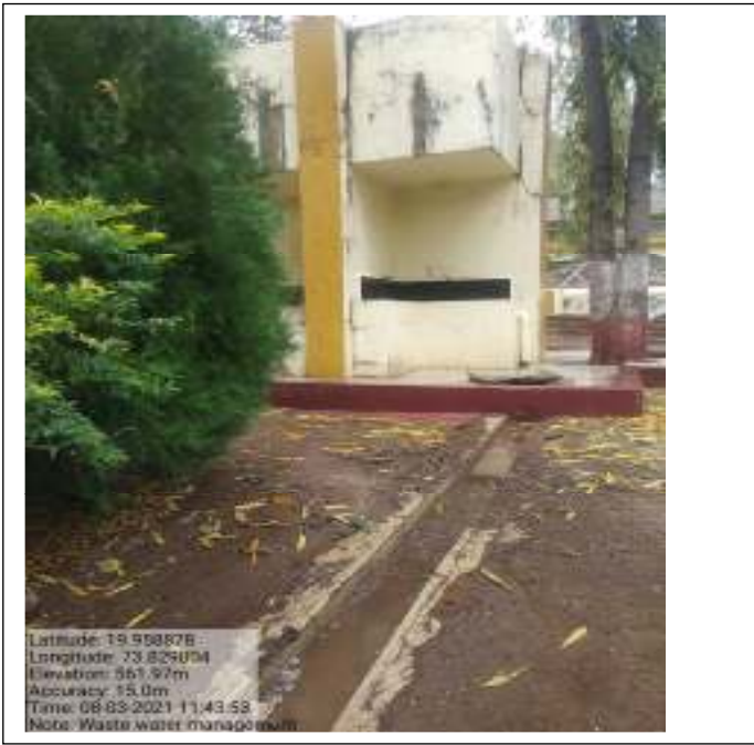
Waste water recycling
